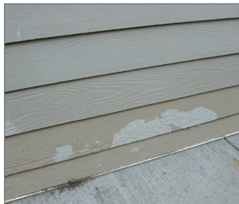
Absorbed moisture can compromise the integrity of fiber cement, causing it to crumble and delaminate.
