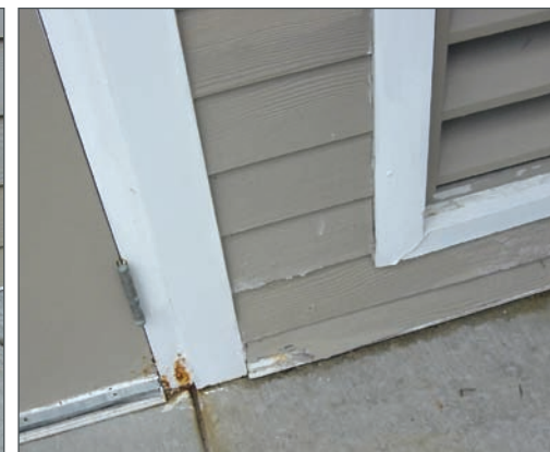
Absorbed moisture can compromise the integrity of fiber cement, causing it to crumble and delaminate.
